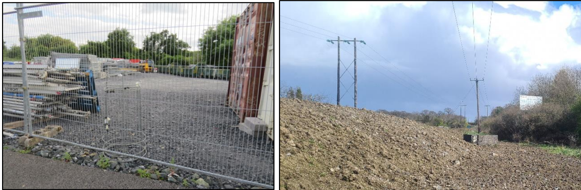
Plate 2: Left - Spoil and bare ground habitat within the campus. Right – haul road undergoing construction in the north lands.
